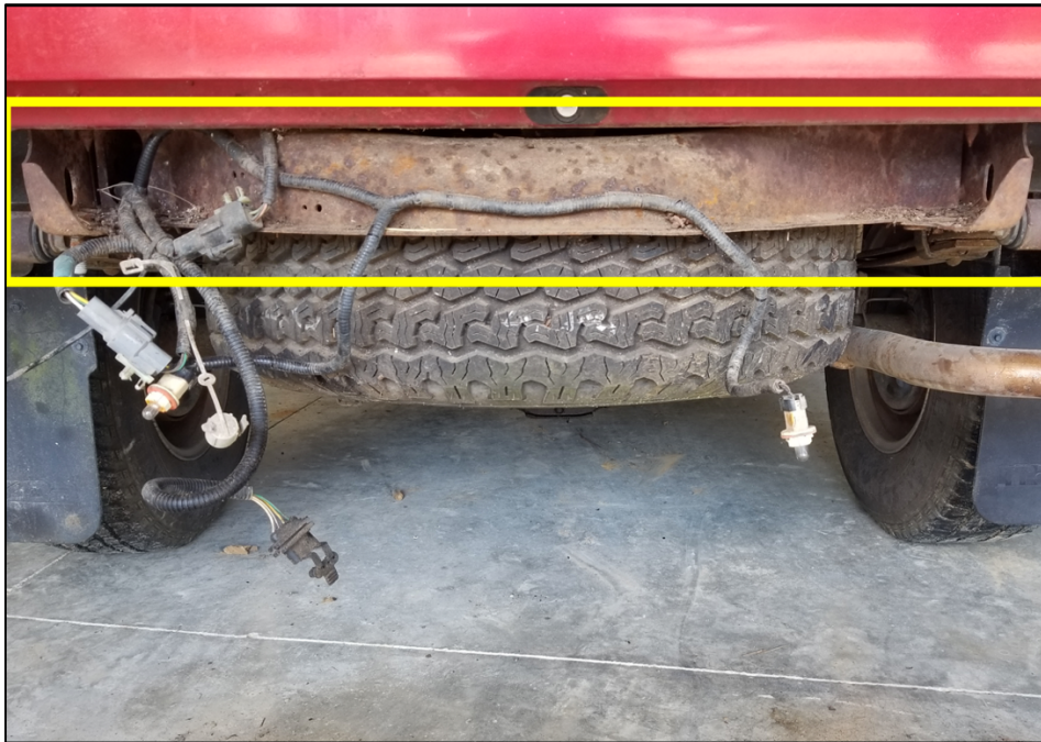
Figure 1. The rear end of the Mazda B3000 pickup truck with the factory bumper removed. The vehicle structure where the interchangeable bumper mount will be attached has been boxed.
